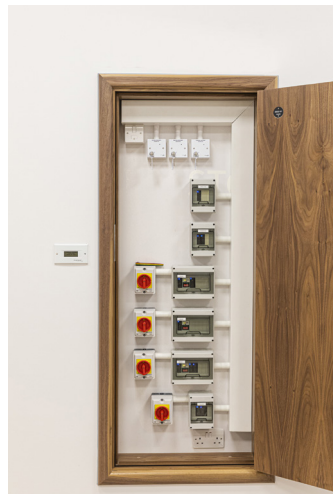
Wide opening for maintenance access
