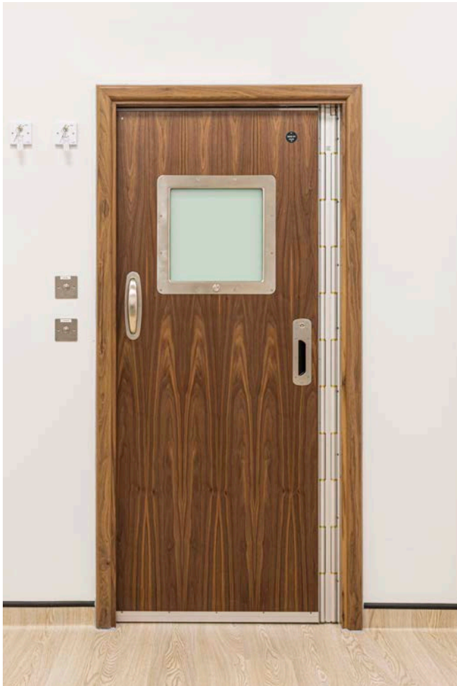
Full height sensor to door edge
