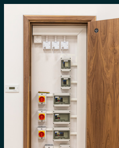
Wide opening for maintenance access
